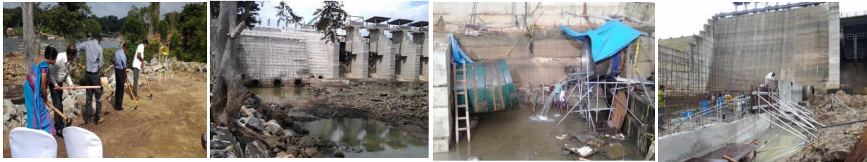
Initiating construction works
