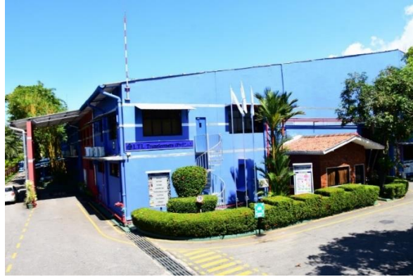
Transformer Plant at Angulana
