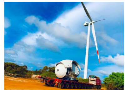
Figure 3: Installation Works of Mannar Wind Power Project
