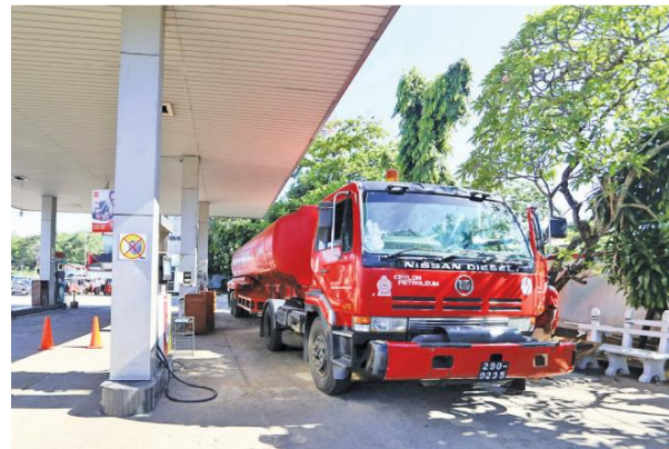
Fuel filling Station
