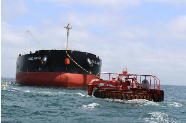
CPC Crude Oil Unloading Buoy
